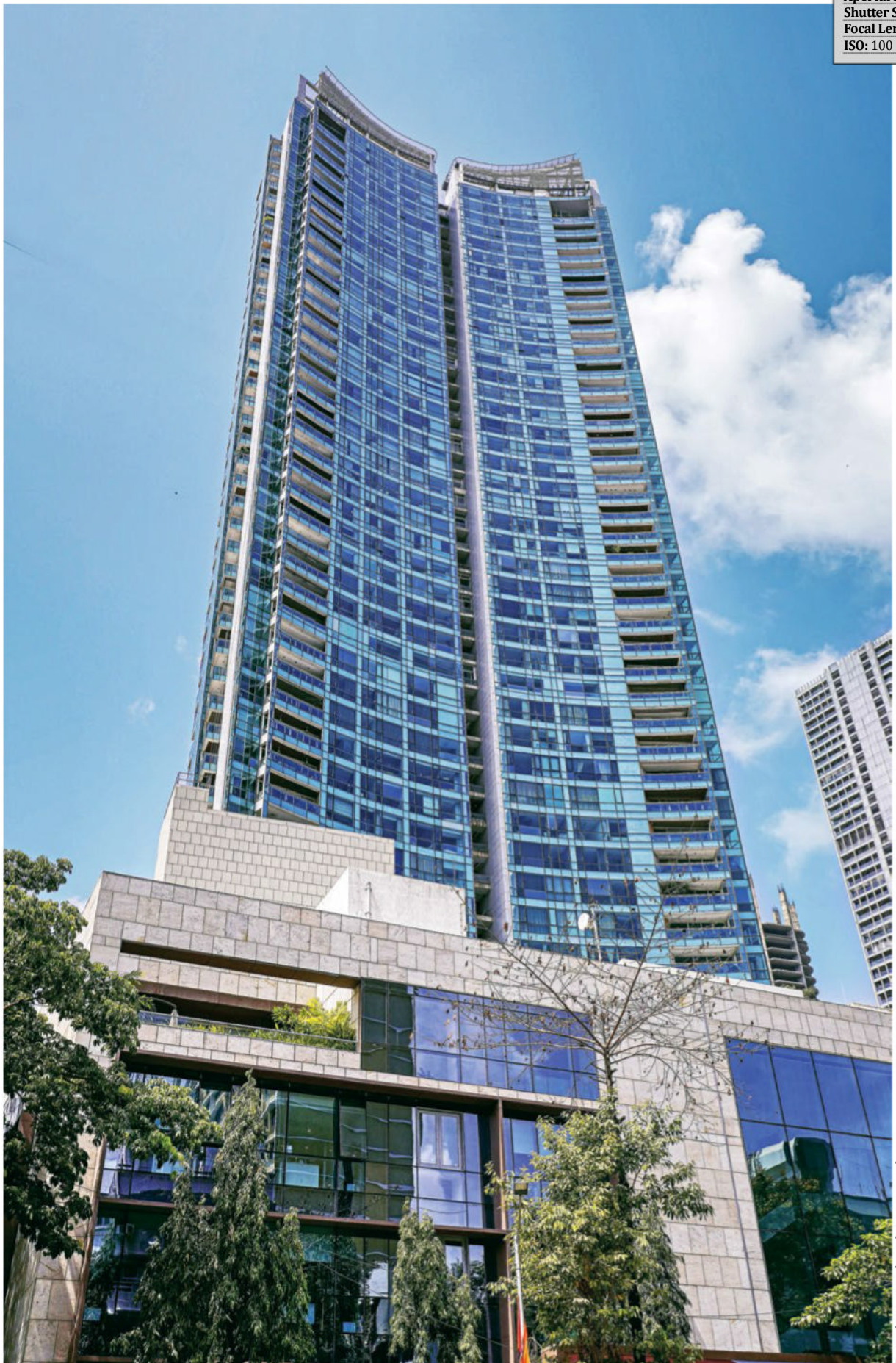
Disturbing wires have been removed.
