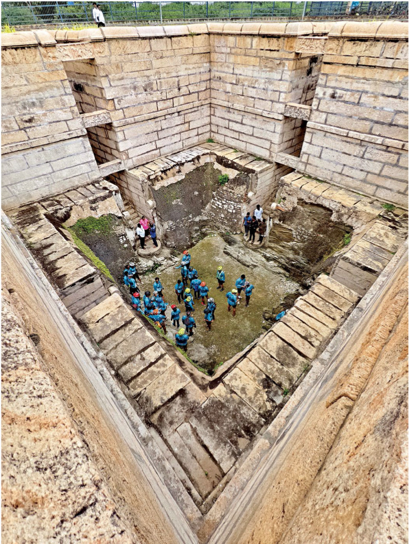
About 22 kilometres from Trichy, behind the temple at Tiruvellarai, sits one of the more quietly remarkable structures in the delta. The Swastika Well, or Marpidugu Kinaru, was excavated in 805 CE on the orders of the Pallava king Dantivarman. Its four arms are cut into the earth in the shape of a swastika, each with 51 steps descending to the water. The geometry is functional. The well was renovated in the 13th century and again in 2013-14
